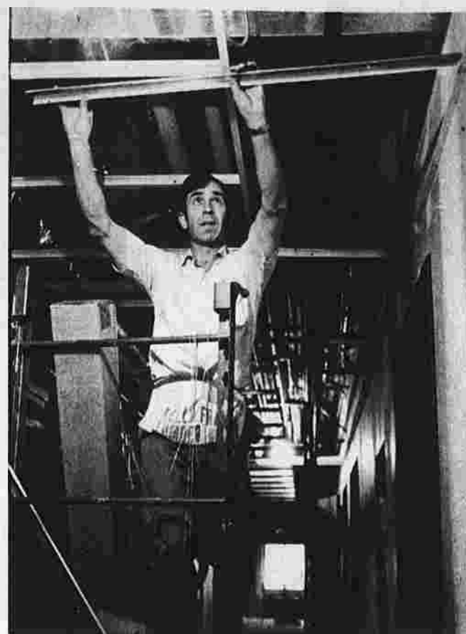
Lenny Bourgojn of Modern Acoustic Co. installs grids for acoustical ceiling panels for construction on third floor of North Wing at Manchester Memorial Hospital.
