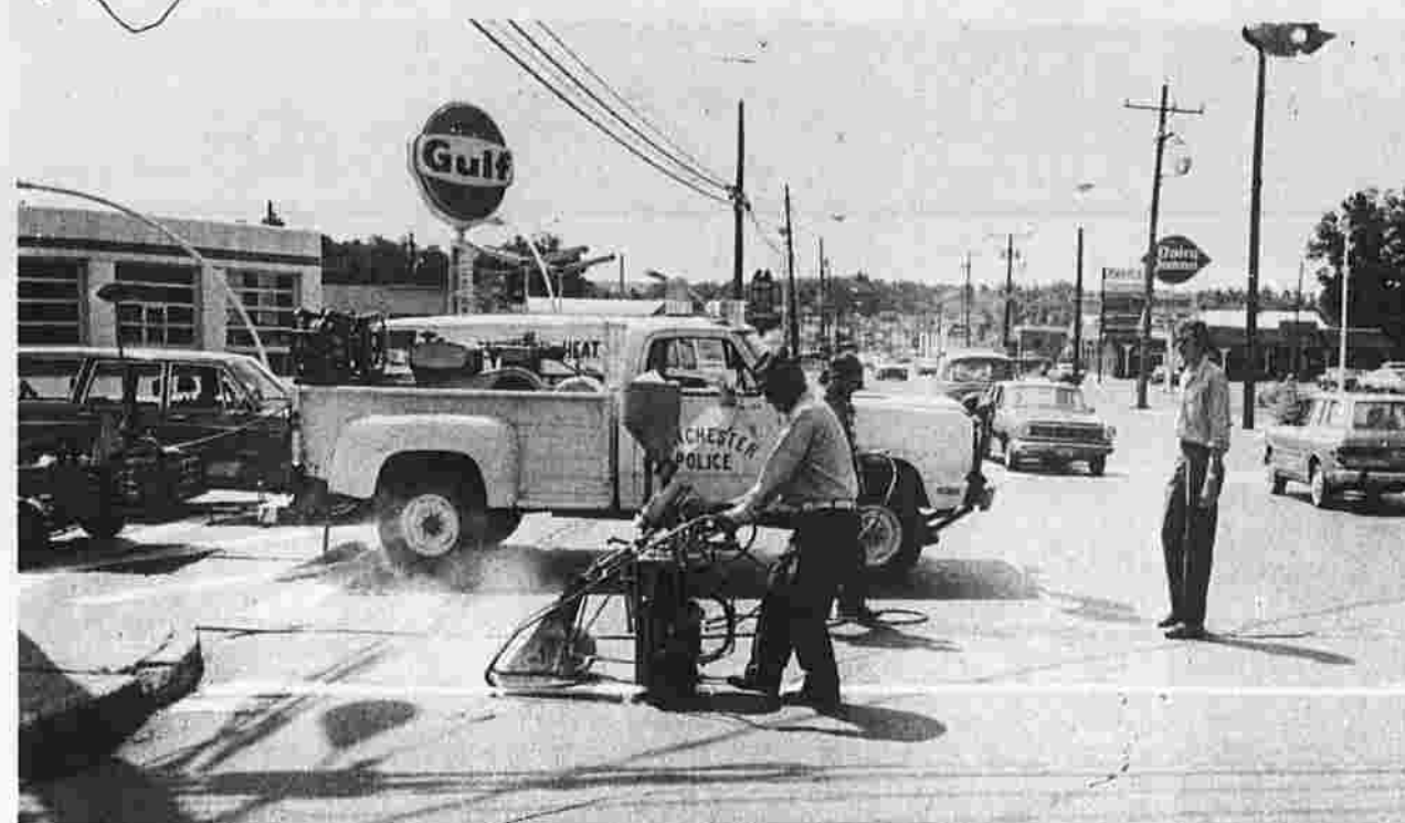
John Evaniski lays down a crosswalk line with a powder paint at Broad St. and W. Middle Tpke. Bob Bagge directs traffic and Phil Byram, a summer youth experience worker, holds the hose.
