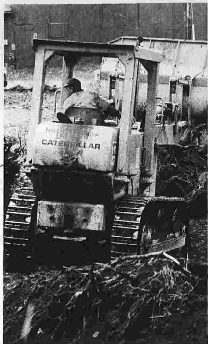
William Burr operates a Caterpillar to clear stumps at the Buckland Firehouse site.
