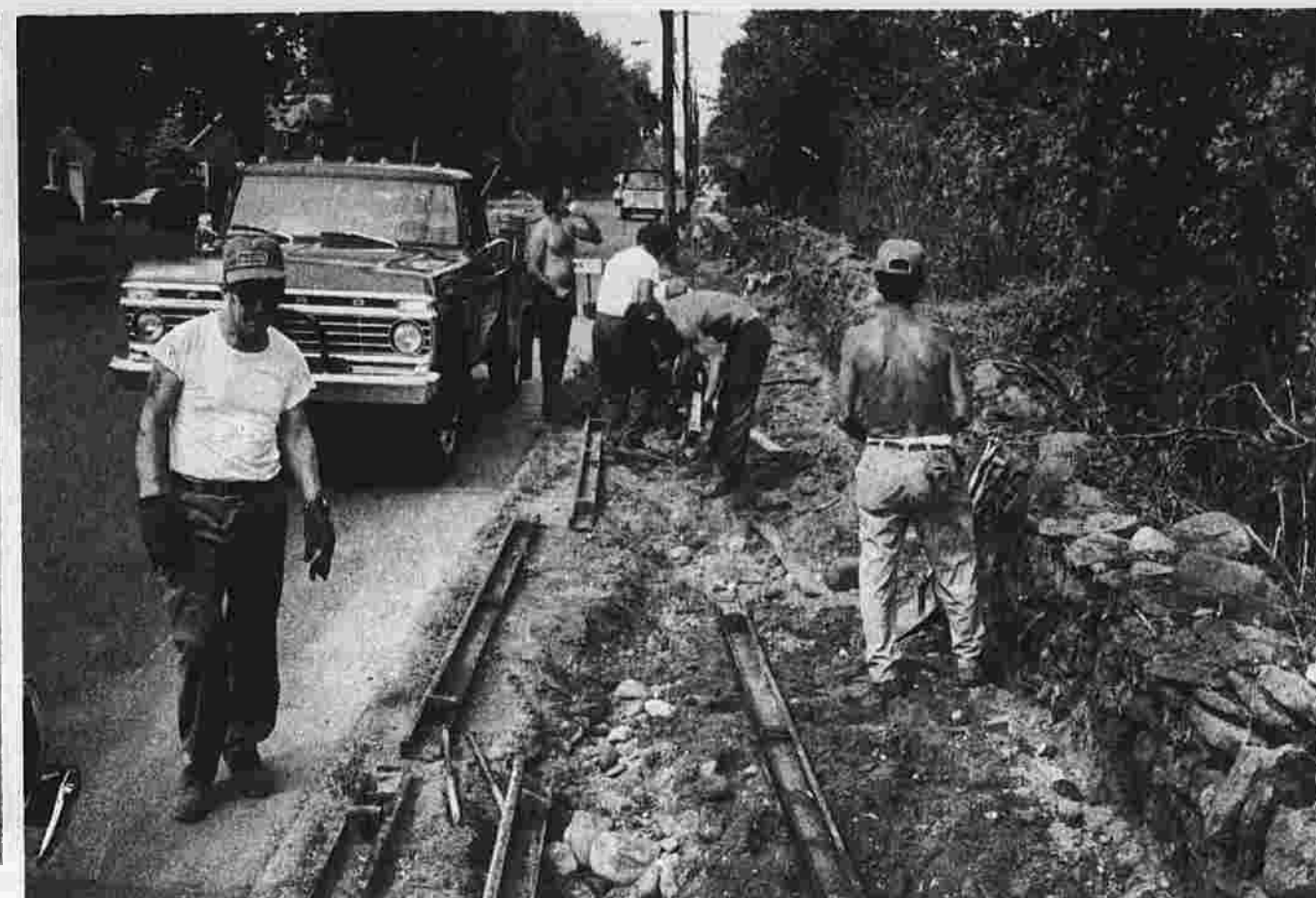
R. Aleria & Sons employees plan the curbing along Oakland St.
