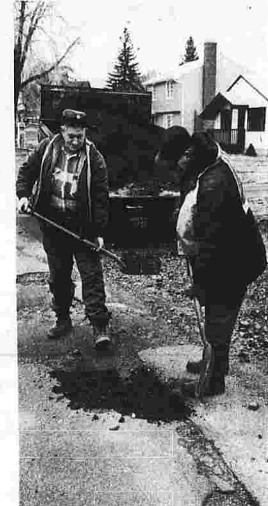
Manchester roads were like other state roads this winter when thaws and floods played havoc with roads. Louis Giglio, left, and Leonard Woodard fill these pot-holes on McKee St.
